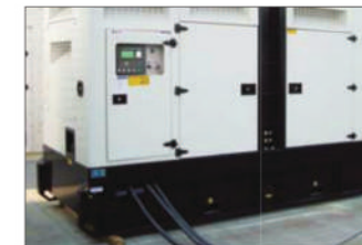
Enclosed power outlet, terminal and sockets
